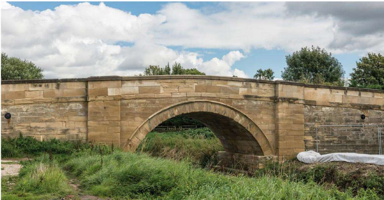
Strensall Bridge: John Carr's bridge
