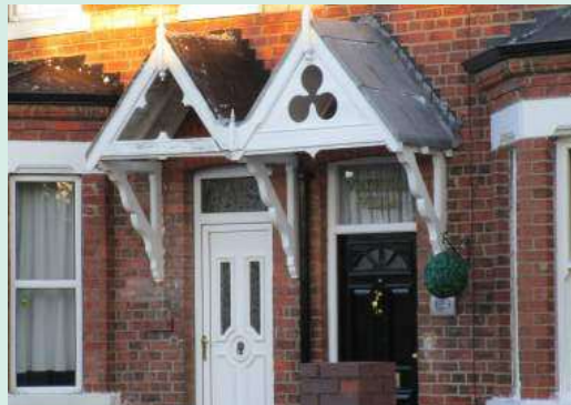
Photo 45: View of decorative detailing
