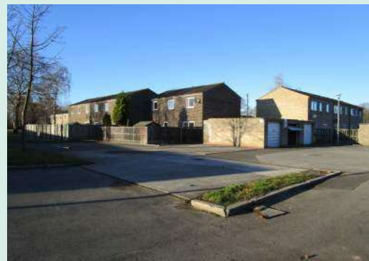
Photo 19: Housing to the north of Howard Road
