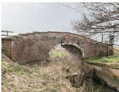
Strensall New Bridge – Haxby Moor Road
