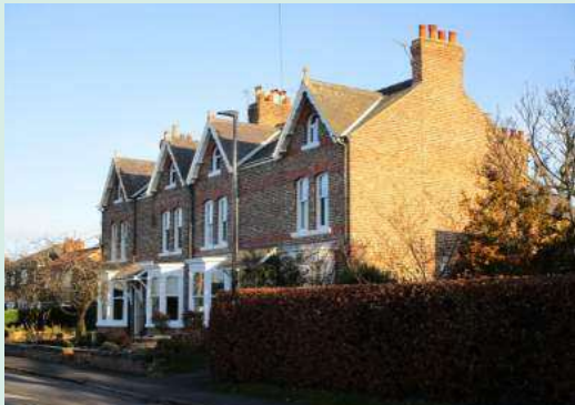
Photo 23: Terrace development with additional rooms accommodated within the roof space
