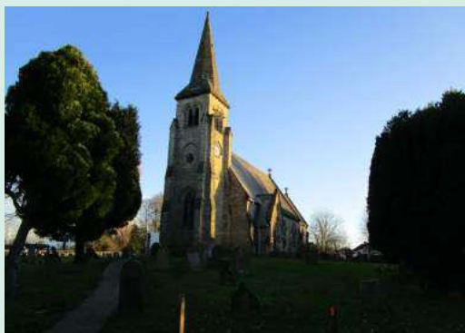
Photo 8: View of St Mary's Church
