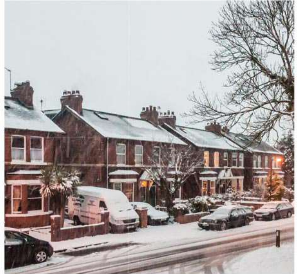
Housing associated with the arrival of the railway in Strensall
