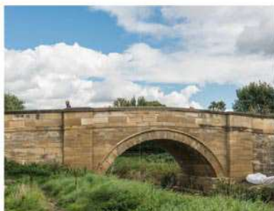
Strensall Bridge – Sheriff Hutton Road
