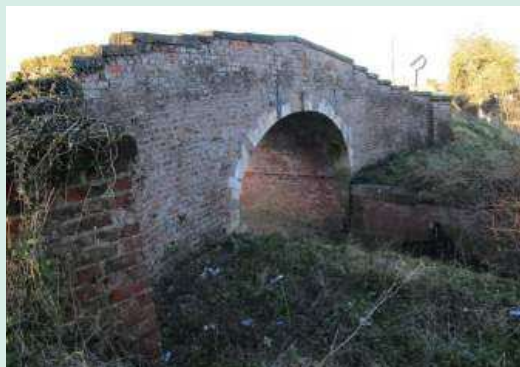
Photo 9: Strensall New Bridge
