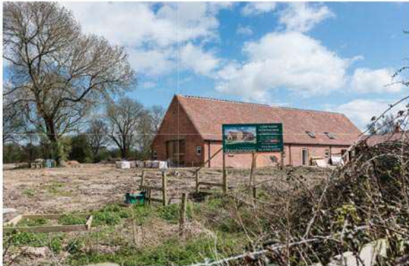
Towthorpe: conversion of agricultural buildings
