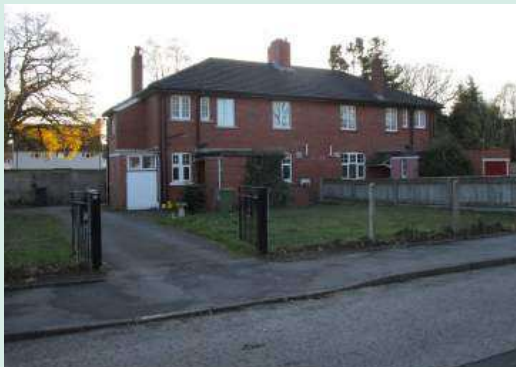
Photo 16: Housing on south side of Alexandra Road
